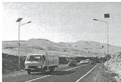
Figure 2: Public highway lightning, Alto Hospicio PV Project.
