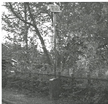
Figure 2: A traffic monitoring unit near Warrington in the North West of England
