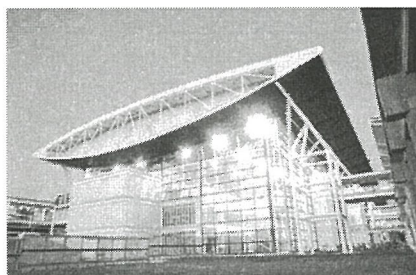
View of the Central pavilion on its early stage.
