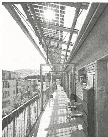
Figure 7: Example of horizontal (canopy) integration.
