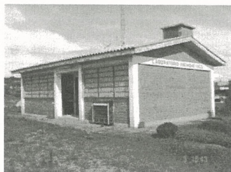
Figure 3 – External view of the thermo-accumulator installed. Source: Own collection
