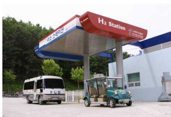
Figure 1. Hydrogen refuelling station at KIER, Daejeon
