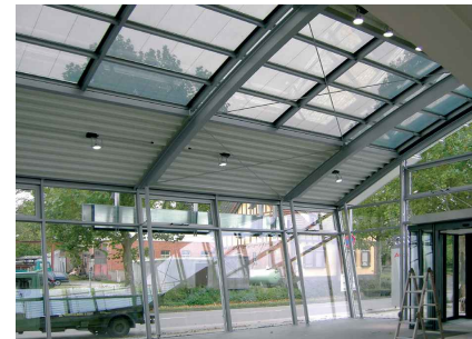
Illustration 6: Roof integrated skylight out of insulation glass components with semitransparent amorphous PV-cells in a showroom in Germany. [Glaswerke Arnold]
