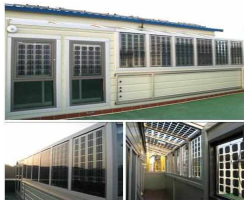
Figure 5: Overview of PV module installation in a sunroom
