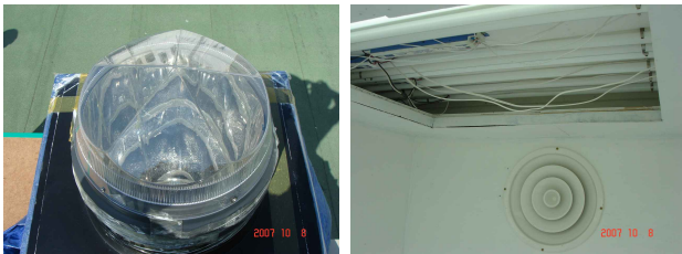
Fig. 3. Sunpipe installed at outside of daylighting chamber (left), fluorescent lamp installed in the artificial lighting chamber (right)
