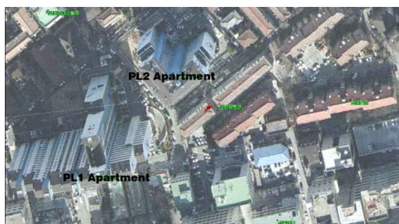
Photo 1: Aerial photo of the PL2 apartment complex before the construction of the SR apartment complex
