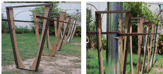
Fig. 4: CPC under construction with parabolic ribs, frames and bracing members.
