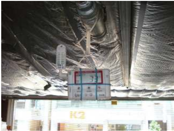
Figure 4: Thermal Recorder for Air current
