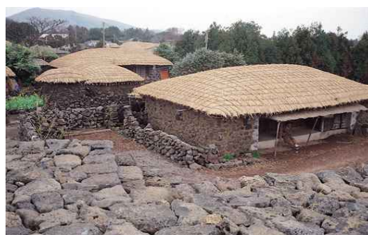
Figure 9. Thatched roof and stone wall
