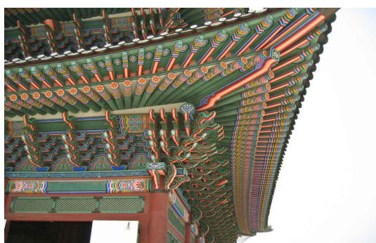
Figure 8. Eaves and rafters
