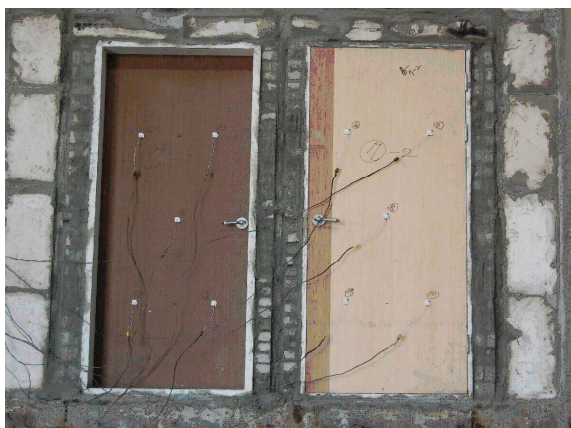
Figure 3: Installed specimen view
