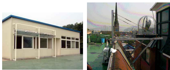
Figure 1: Sun deflectors and sun lighting system developed by the authors (at Kyung Hee University).
