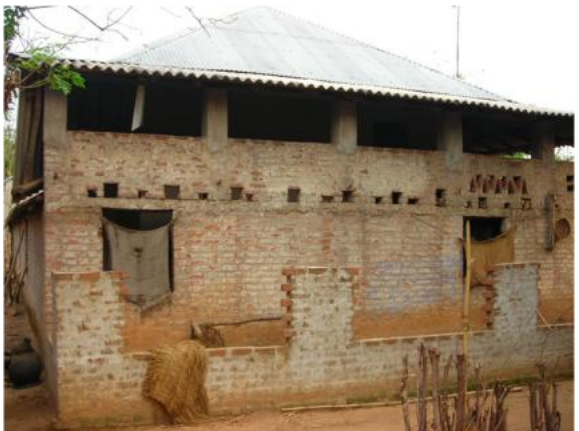
Figure 5: Transition Phase 3: tribal shelter with burnt-brick walls in cement mortar and tin roof (replacing earthen walls and thatch roof)
