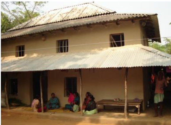
Figure 3: Transition Phase 1: tribal shelter with tin roof (replacing thatch roof)
