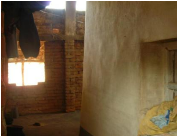
Figure 4: Transition Phase 2: tribal shelter with burnt-brick walls in mud mortar (replacing earthen walls)
