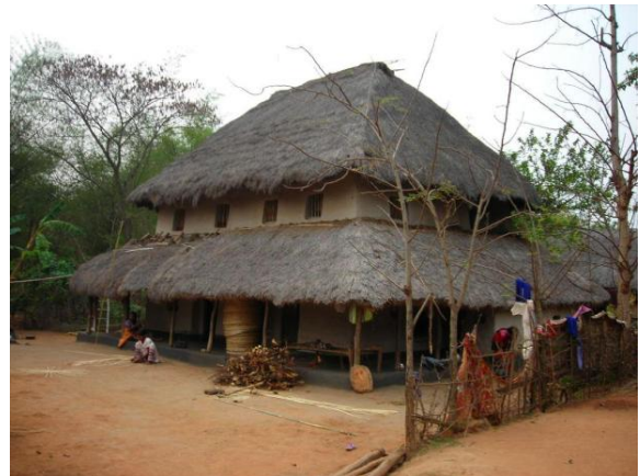
Figure 2: Traditional Two-Storied Tribal Shelter (earthen walls, thatch roof)
