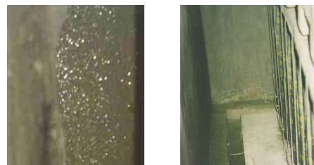
Figure 2: Condensation in Igloo magazine
