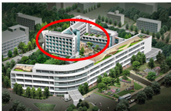
Fig 1: Building of the ground source heat pump system installed.
