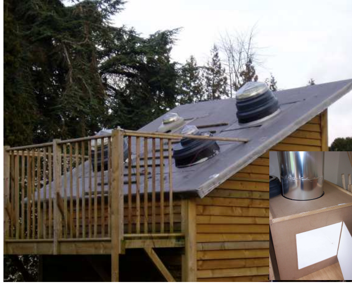
Figure 1: The purpose built Monodraught test shed at the School of the Built Environment, University of Nottingham
