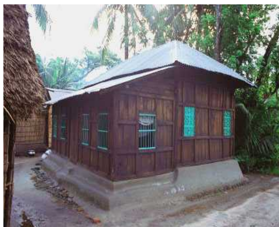
Figure 4: Timber wall house [5]
