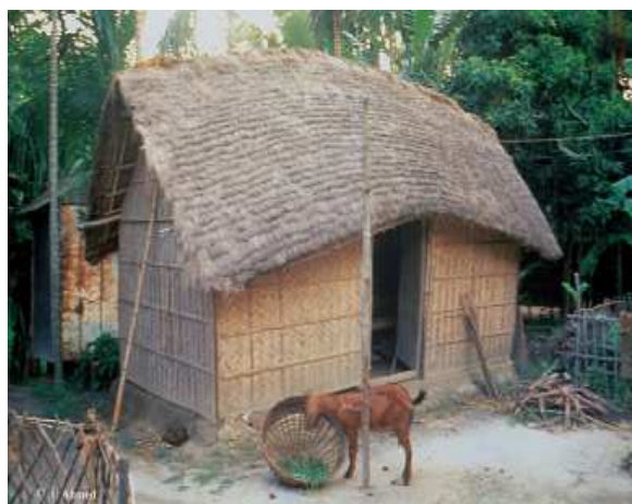
Figure 2: Bamboo wall house [5]
